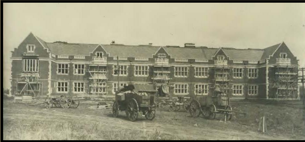
Reed College, Eliot Hall, under construction, 1911
