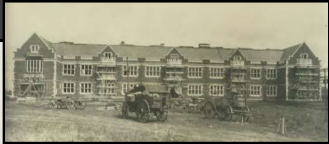
Eliot Hall, under construction, 1911
